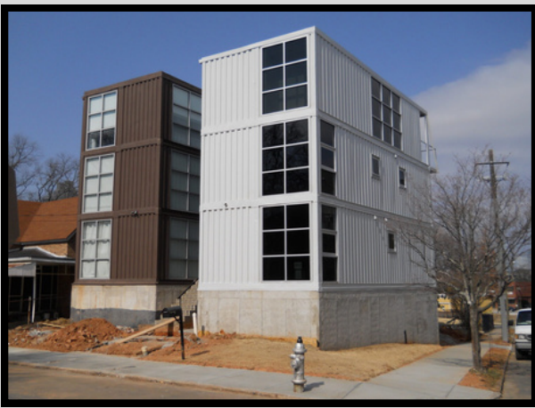
Our first two shipping container homes, built in Atlanta in 2008, were the first of their type built in Georgia.
