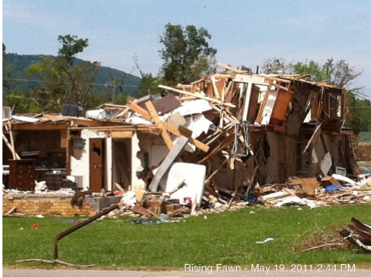
Tornado damage near Trenton, GA from the April 2011 tornado (an EF-4 tornado)
